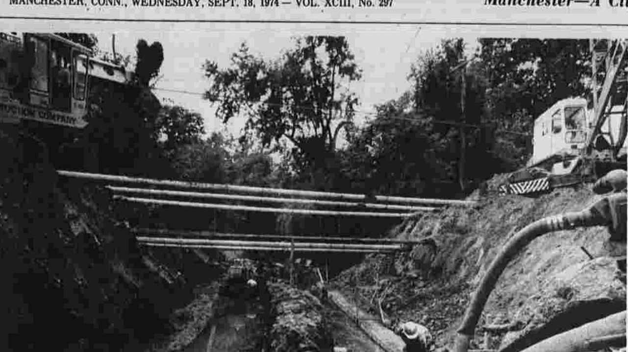
Woodbridge St. Bridge Work Under Way
